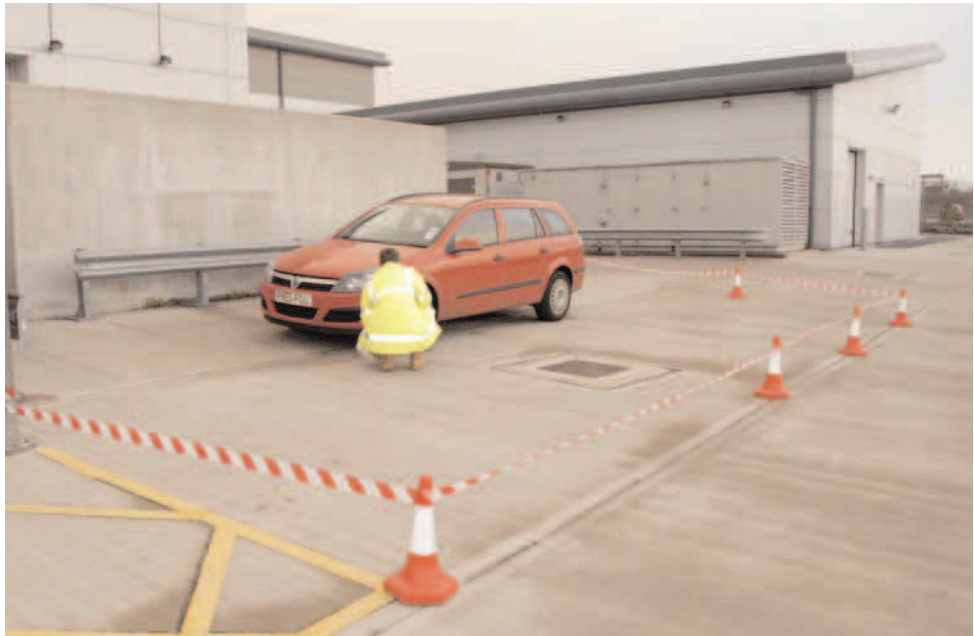
Figure 8 Spraying outdoors in a cordoned-off area
